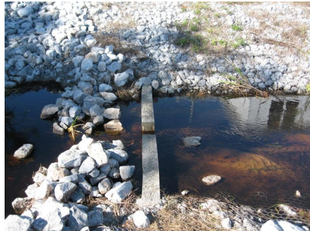
b. Completed Weir Structure Used to Provide Constant Control Section for Flow Measurement
