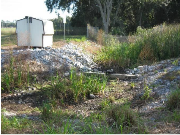
a. Equipment Housing for Inflow Monitoring Site
