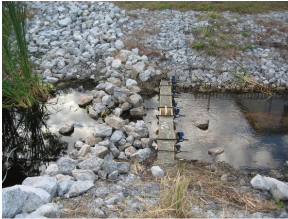
a. Weir Structure formed and Poured with Concrete
