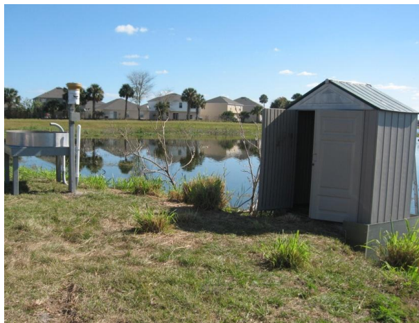
a. Hydrologic Monitoring Equipment Adjacent to Outfall Structure
