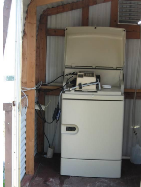
b. Refrigerated Autosampler Used for Inflow Monitoring
