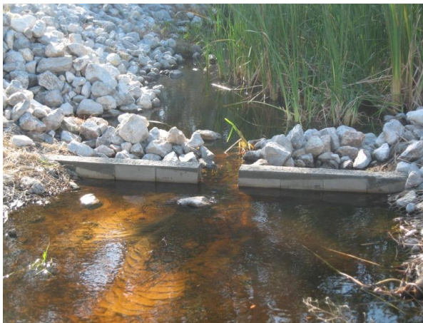
b. Completed Weir Structure Used to Provide Constant Control Section for Flow Measurement
