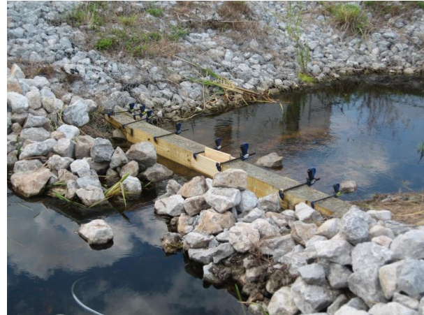
a. Weir Structure formed and Poured with Concrete
